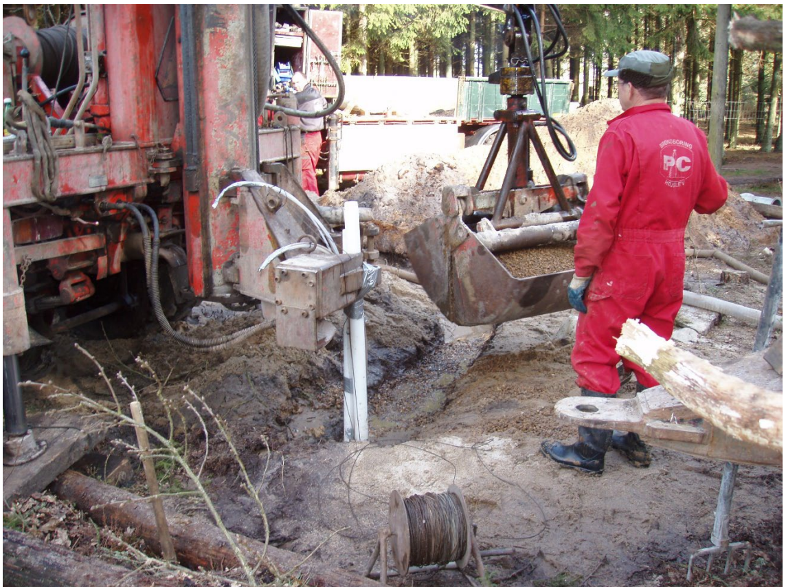
Figure 1. Well completion. In this case, there are two casing strings in the same borehole.
