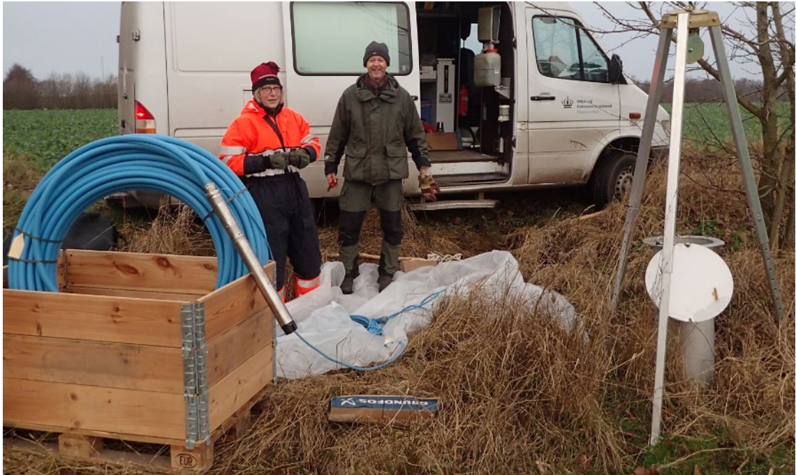
Figure 7. Preparation for installation of a larger electric submersible pump and hoses. The equipment is pre-assembled in the workshop, where hose lengths are adjusted to the technical completion of the borehole.
